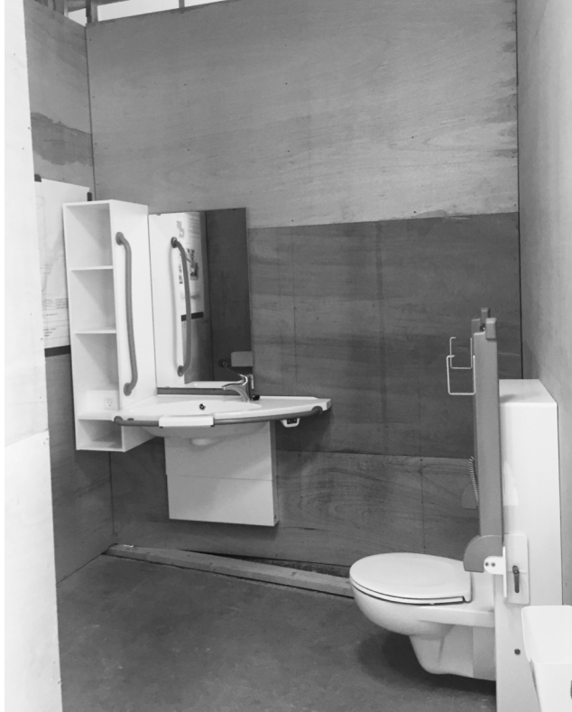
Figure 4. First version of the mock-up of standard patient bathroom that will become a fully functional patient room for ‘embodied reviewing.’
